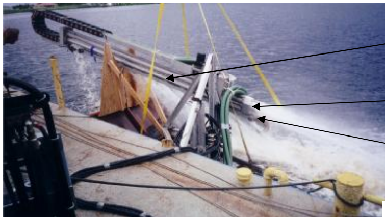
DeepGrab Jetting System Shoreside Trials
